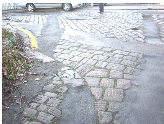
58. Surviving setts in Well Meadow Street - typically laid obliquely to the road line.
