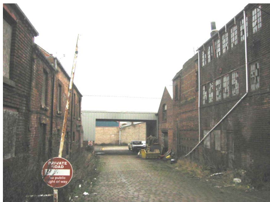
60. Looking north-east along Well Meadow Street.
