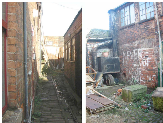
75. Courtyard spaces to rear of 52-56 Garden Street.
